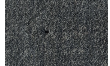
Example of blowhole (enlargement).
